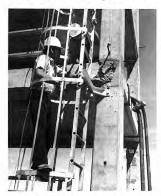
BUILDING INSPECTORS Hank Passmore (1131), left, and D. Ellett (1150) check damage to third-floor joint after NTS building shake test. Hank assisted in providing test site logistical support; D. was test director. Note spalled concrete and bare re-bar. (Photo by Pan-Am)
